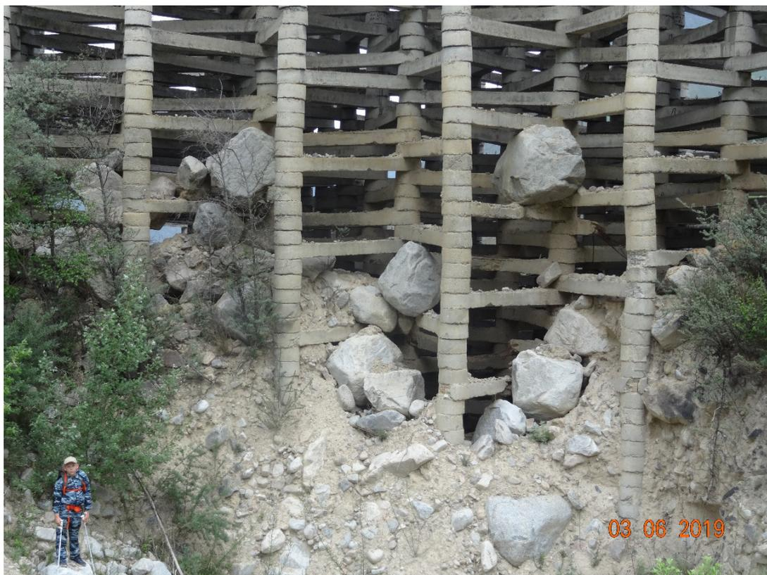
Fig. 11. Blocks of the rocks up to 1.5 m in diameter, lodged in the semi-permeable dam on the altitude 2–4 m
